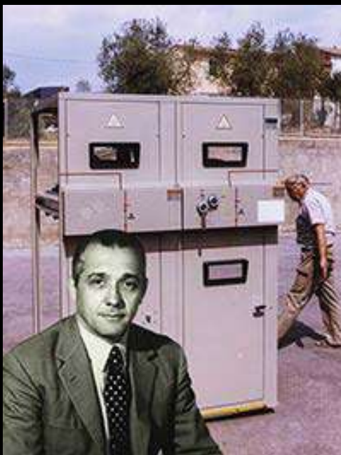
Giorgio Leporatti while is inspecting a M.V. Switchboard
